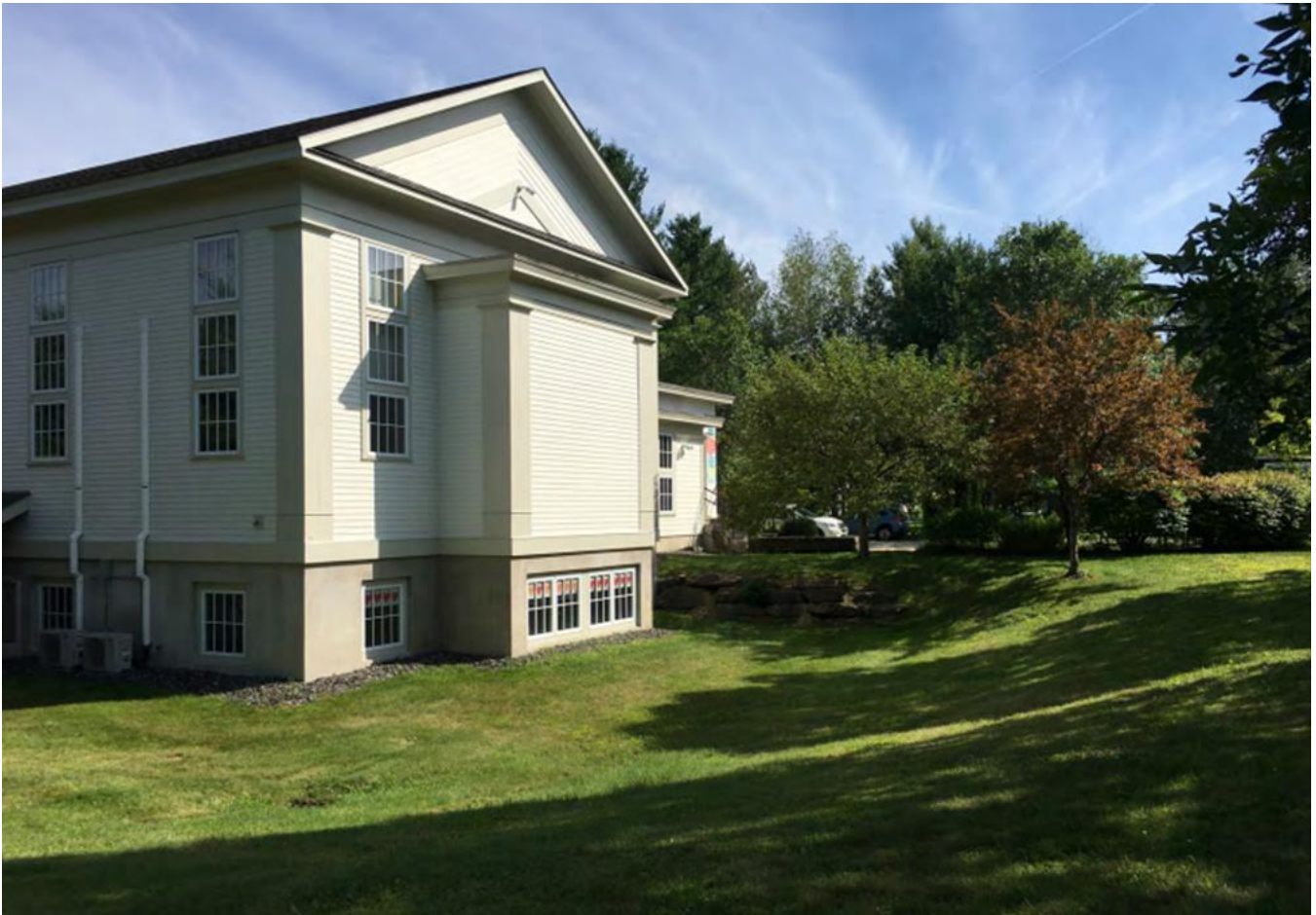
9. The site, looking southwest.
